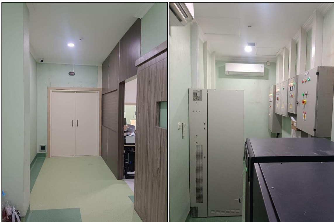
Gambar 7 Rehabilitasi Ruang Cathlab
