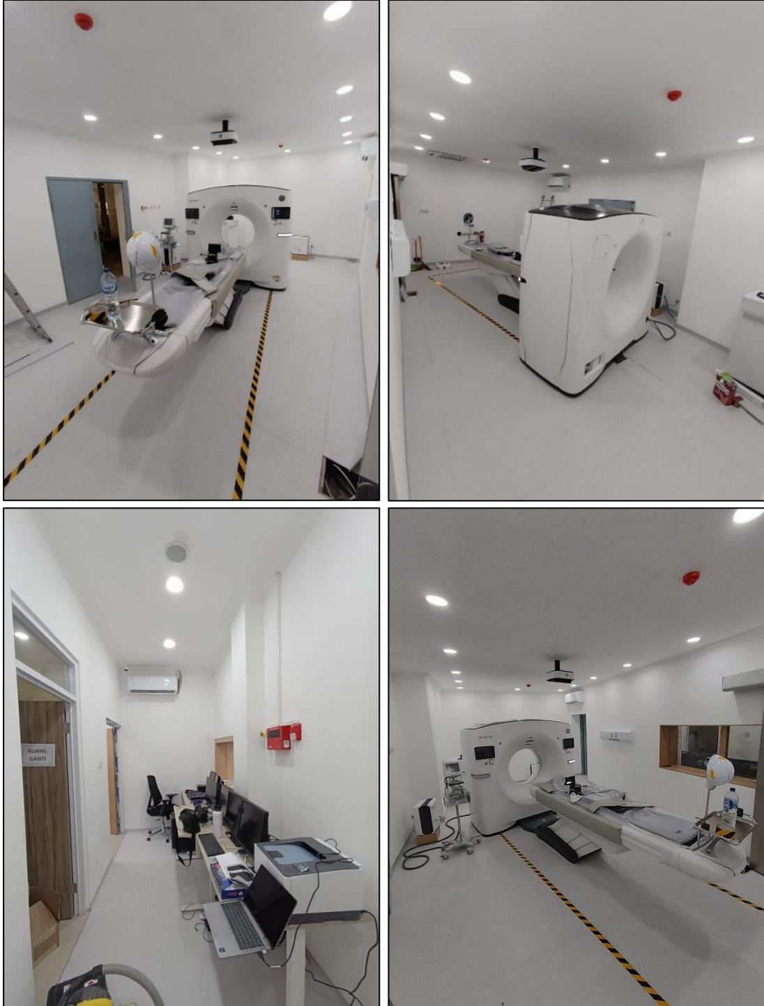
Gambar 6 Rehabilitasi Ruang CT SCAN
